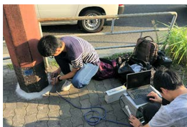
Fig. 1 Inspection of underground corrosion at a road marker pole.
